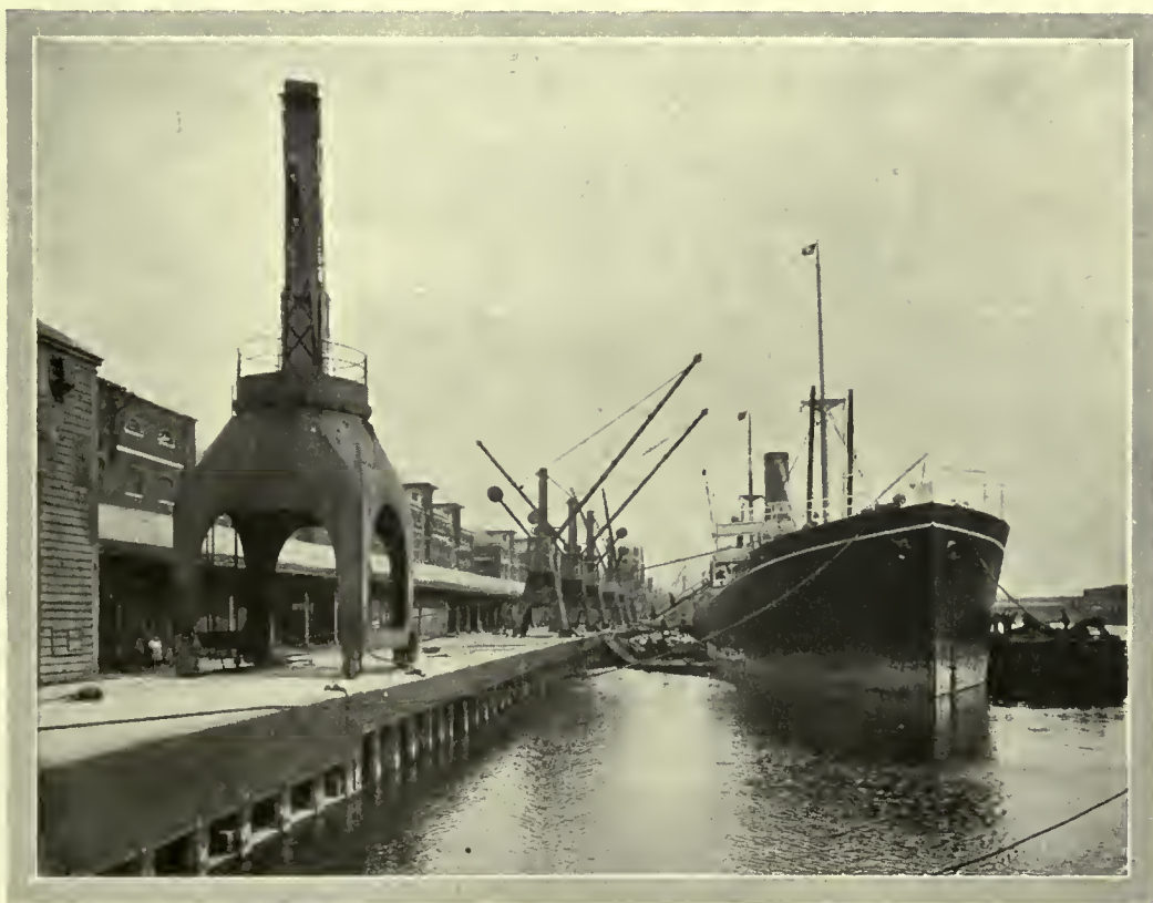
TRAVELLING CRANES IN A LONDON DOCK.
