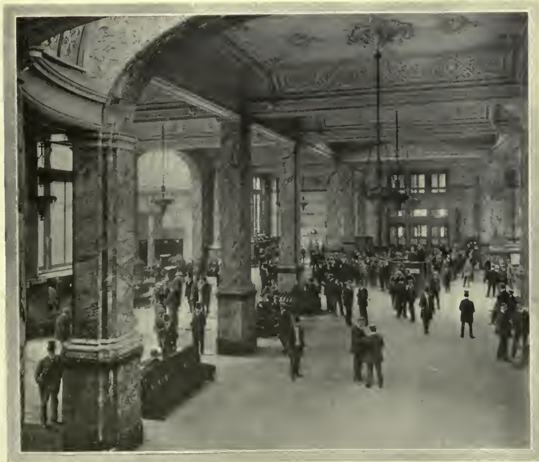
THE MARBLE HALL AT THE BALTIC EXCHANGE.
