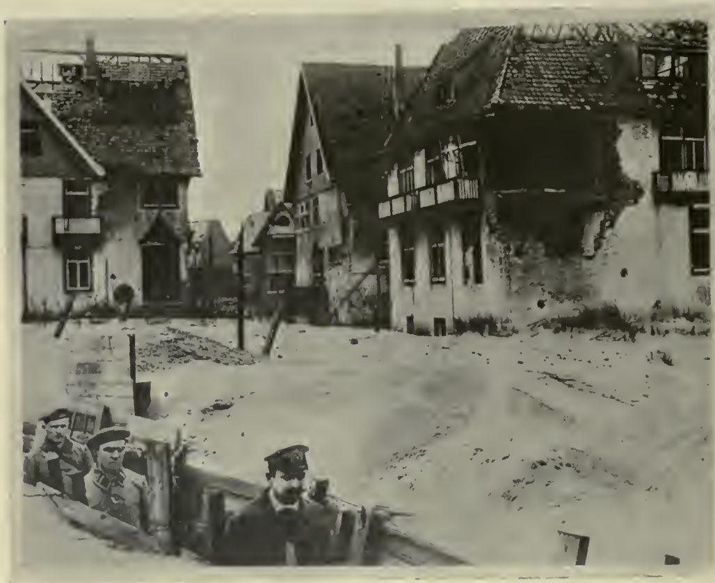
TRENCH DUG BY THE GERMANS THROUGH A FLEMISH COAST VILLAGE.
