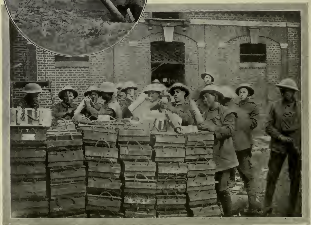
FITTING FUSES TO STOKES BOMBS.
