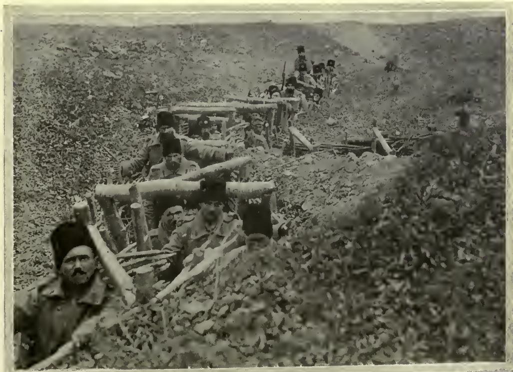
A COMMUNICATION TRENCH.
