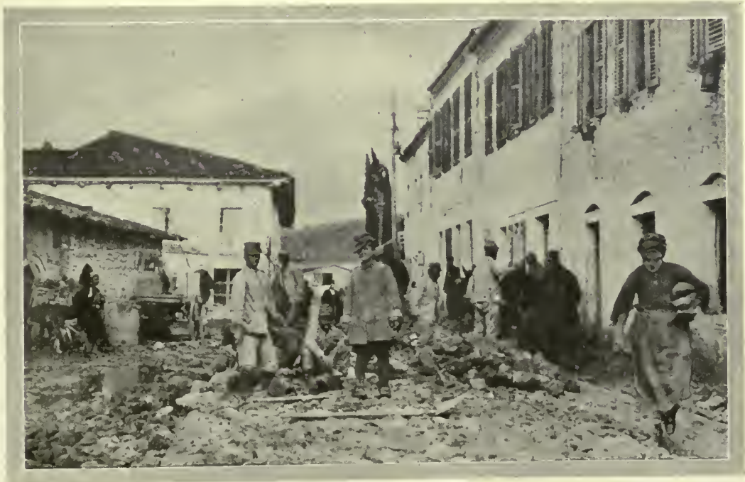
ITALIAN RESERVISTS REPAIRING ROADS IN VALONA.
